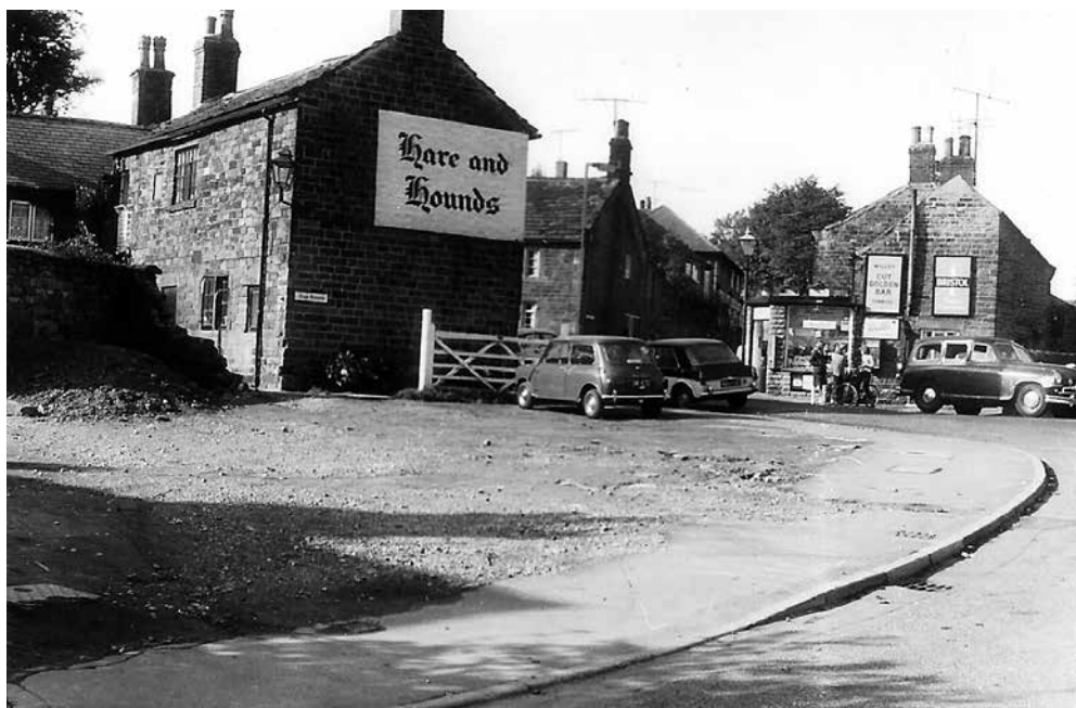
The Hare & Hounds before the attached shops were demolished, and Jester's Cottage when it was still a shop. The cottage which stood in the foreground had only just been pulled down in 1964, and is now the outdoor seating area.
