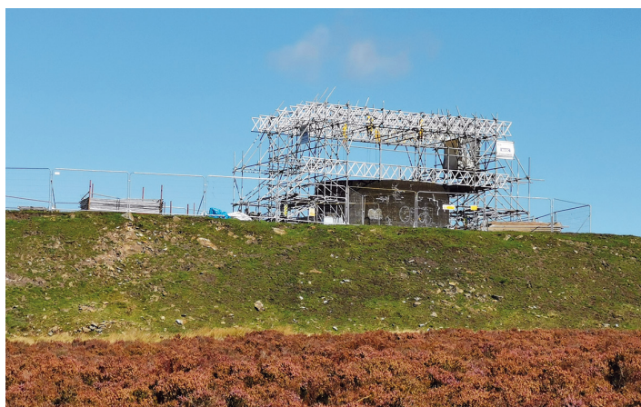
Work on the air shaft on Totley Moss.
