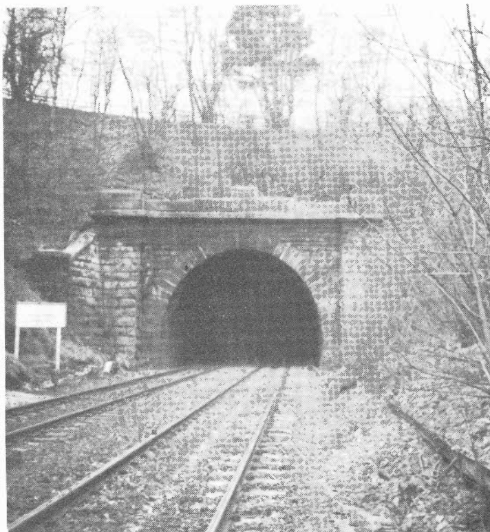
Entrance to Totley Tunnel
