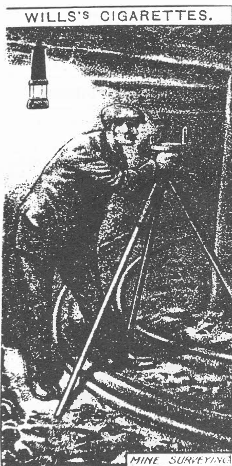
Cigarette card published 1916 showing a mine surveyor "dialling" bearings underground.
