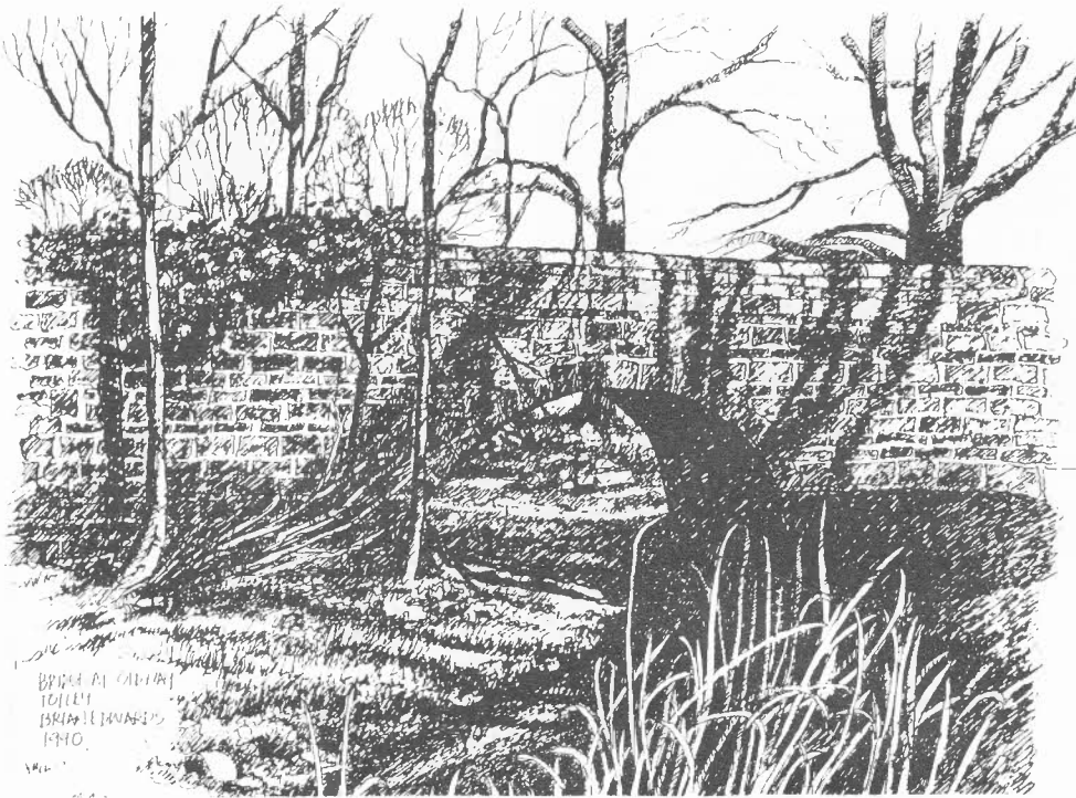
Bridge over Old Hay Brook on Old Hay Lane. An illustration for Brian Edwards new book Sheffield and the Peak .
