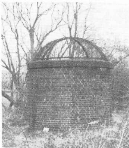
One of the typical peppertop tops to ventilation shafts on the tunnel.
