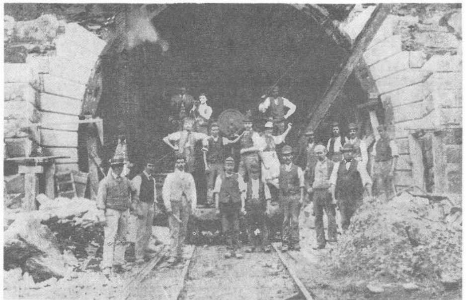
Construction of the Totley Tunnel East entrance. See letter and centre feature in our last edition.
