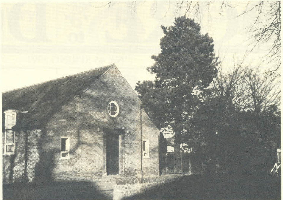
Trees in the electricity sub station adjacent to the church hall on Townhead Road.
