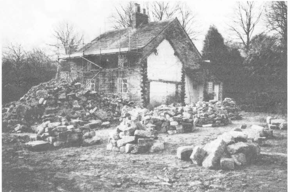
Nab Farm January 2000. All that was left after demolition.
