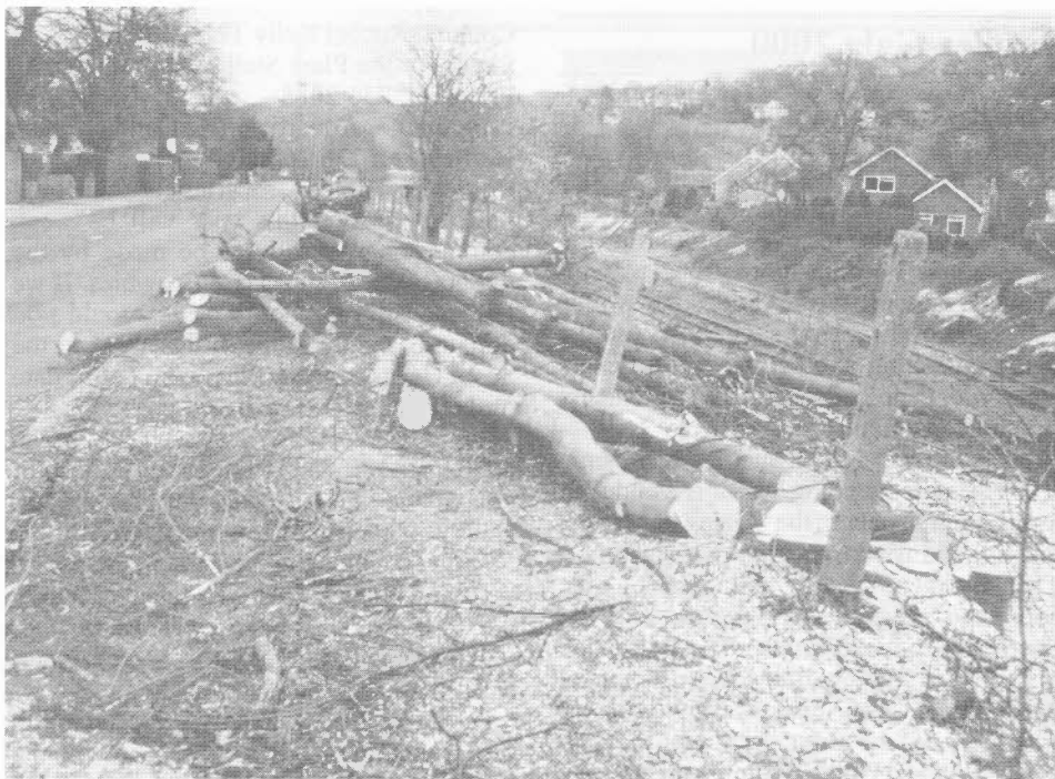
Devastation on Totley Brook Road after contractors working for Railtrack fell all the mature trees on the embankment.
