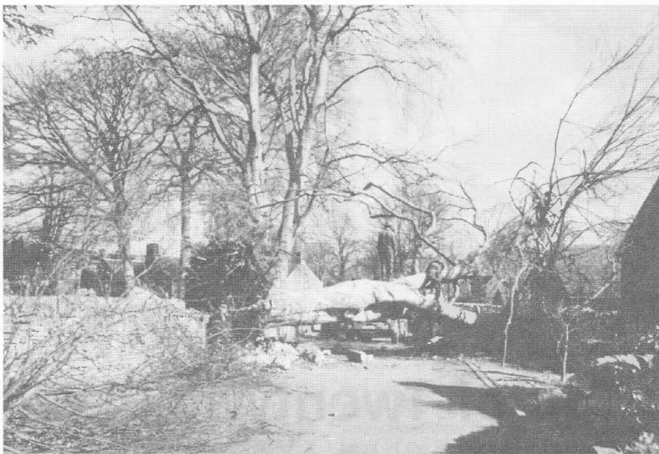
Above: Council workmen begin removing the tree which blocked Vicarage Lane.
