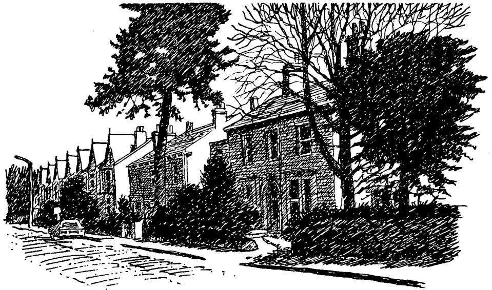
Victorian houses on Abbeydale Road South.
