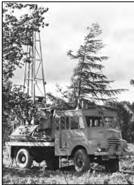
City of Sheffield Estate Surveyor's drilling rig, on the site of the proposed Rushley Road estate. Graham Thomas
