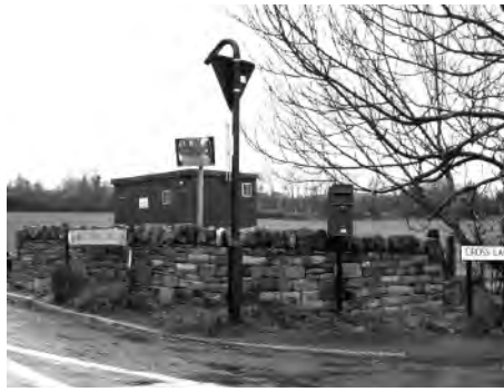
Congratulations to National Grid for constructing a very handsome dry stone wall in front of their new metering station at the junction of Brickhouse Lane and Cross Lane.
