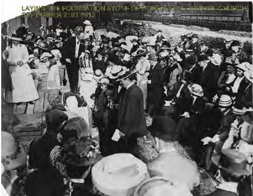
Laying of the URC foundation stone in 1912. Photograph published with permission of the Dore & Totley United Reformed Church Elders
