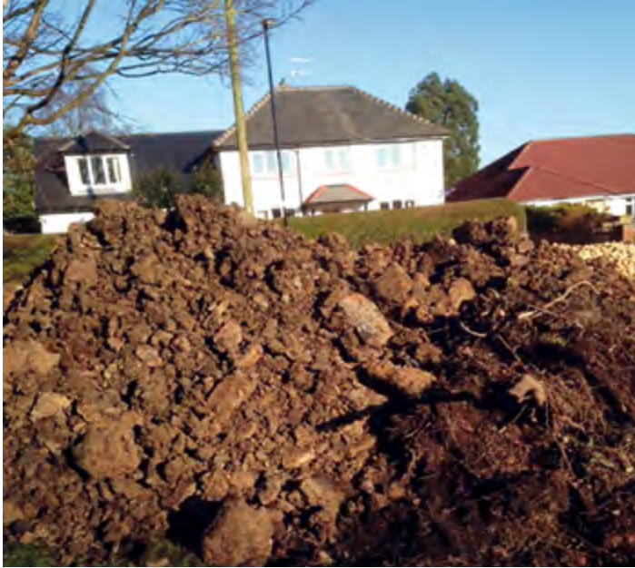
Not a pretty sight - piles of earth over the planted verge at the junction of Causeway Head Road and Parkers Lane
