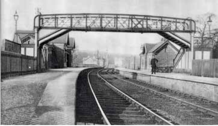
Dore & Totley Station 120 years ago. Two brick-built waiting rooms, though the trains were cold and draughty
