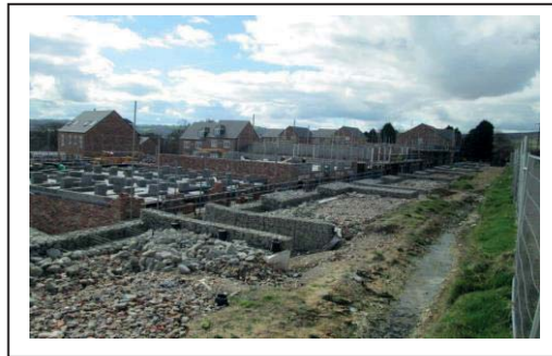
Housing under construction at Wyvern Grange
