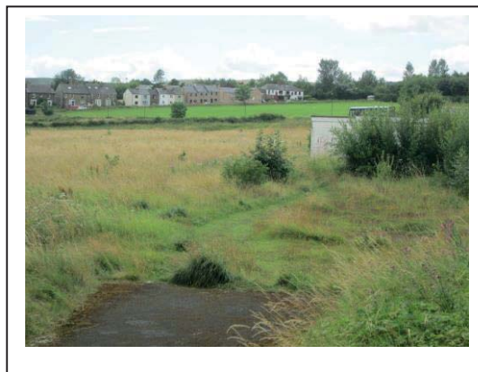
Derelict Sports Pavilion off Cross Lane
