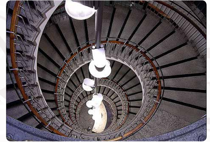
Castle House to be refurbished as Tech Incubator – main staircase detail
