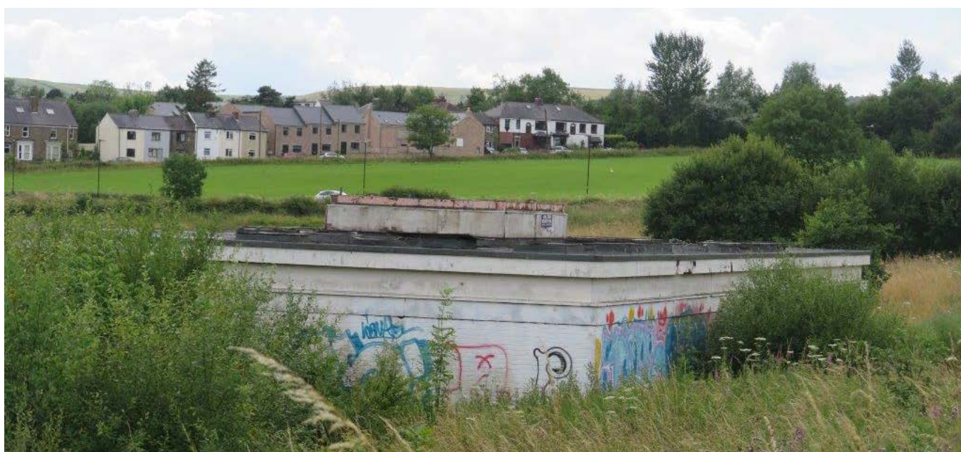
Derelict Sports Pavilion off Cross Lane
