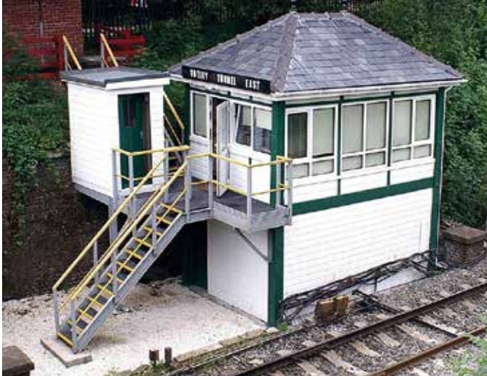
Topley Tunnel East signal box
