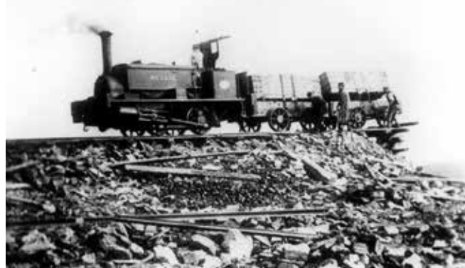
Steam Locomotive 'Nellie', used during the construction of Topley Tunnel - © PictureSheffield.
