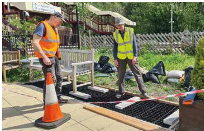
New benches being installed in the pick-up area, made possible by donations from FoDaTS and Abbeydale Rotary.
