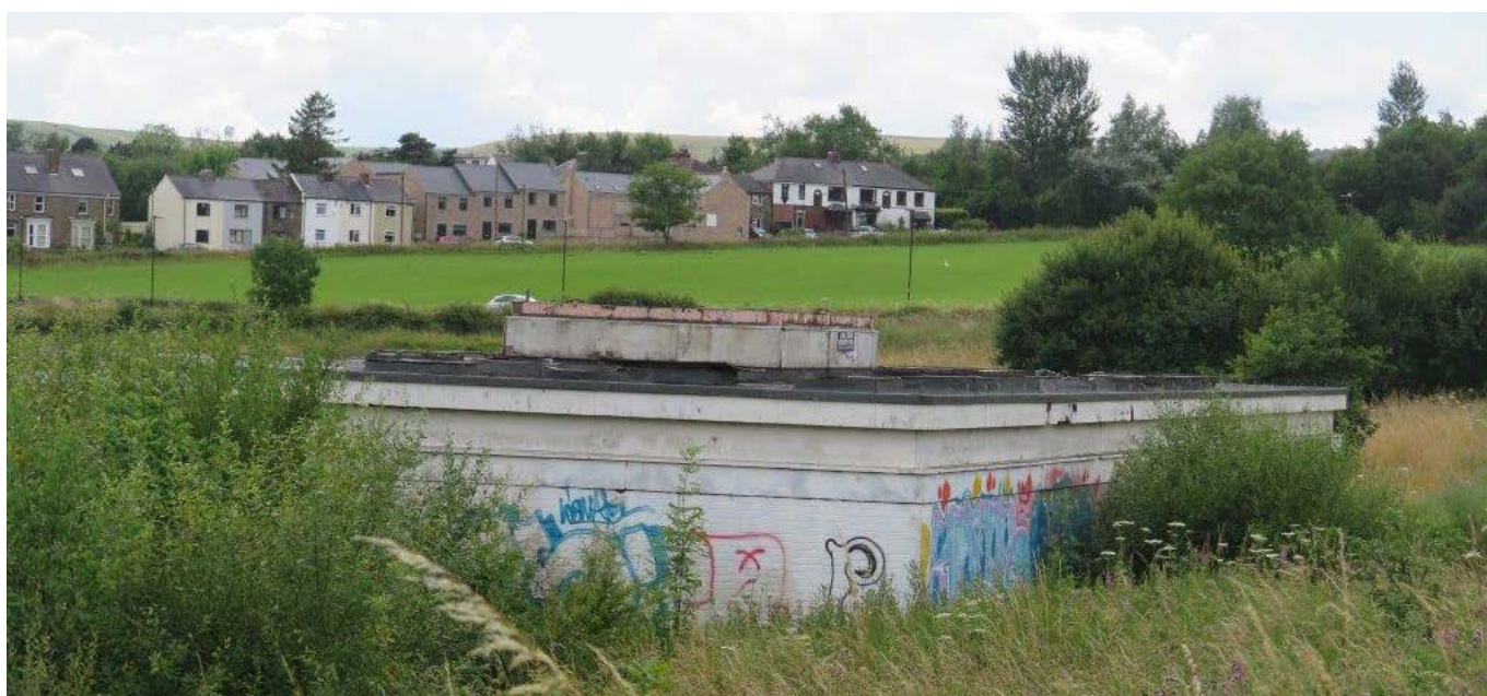
Derelict Sports Pavilion off Cross Lane
